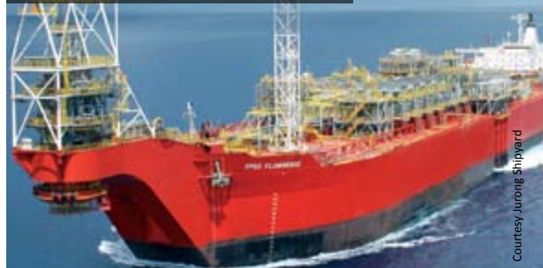
Water Injection Pumps, Gas Compressors & Fire Fighting Pump - FPSO Fluminense - Shell, Brazil
