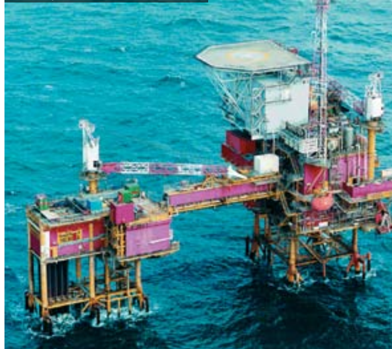
Oil Pumps - Helder A - Shell, Nederland
